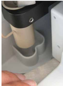
Fig. 40: Drying the leak sensor
